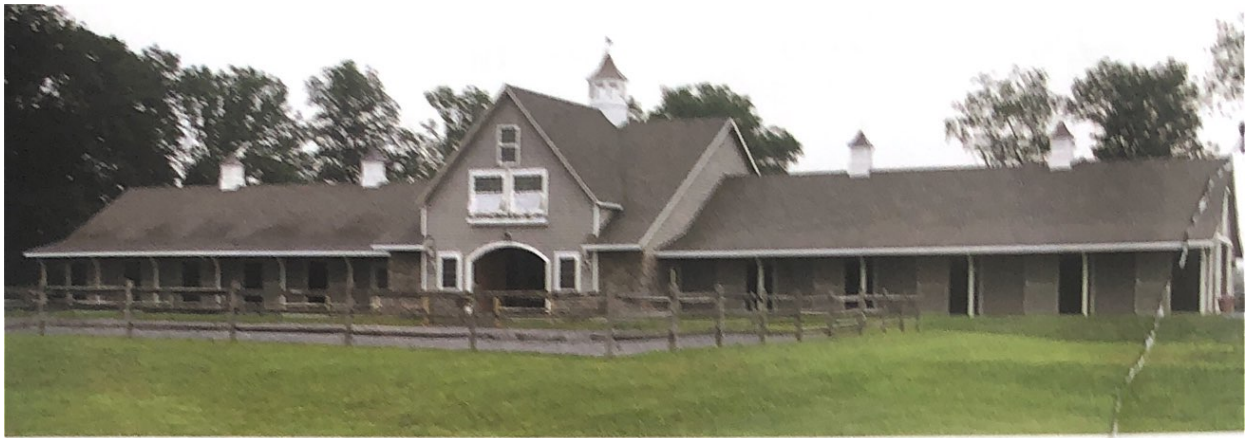
The barn at Thornewood Farm in Stockton, NJ, has been expanded from nine to nineteen stalls
